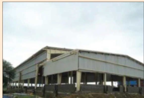
General Storage Bldg.
