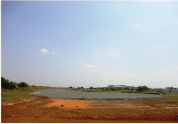
3. Braking Surface Track
