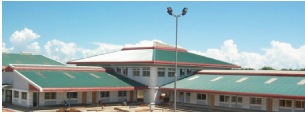
Canteen & Guest House Building
