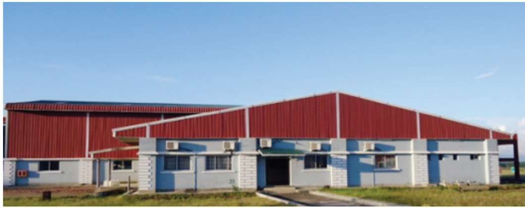
Inspection & Maintenance Station (IMS)
