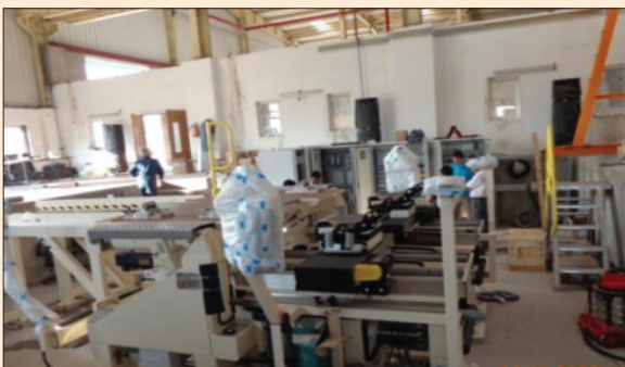
K&C Machine under installation
