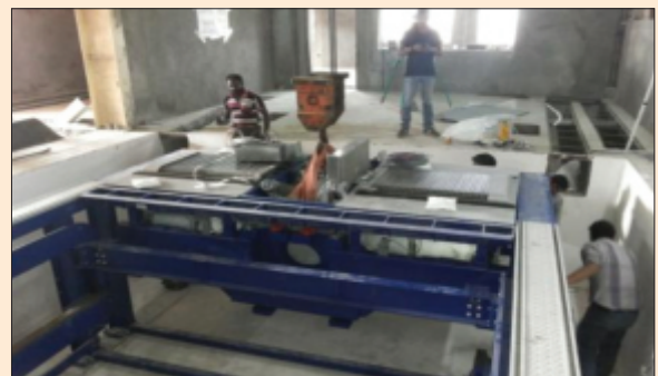
Chassis Dynamometer under installation
