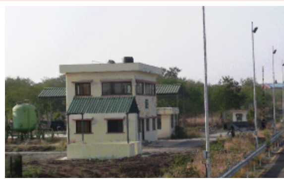
Control Room with Water Treatment Plant
