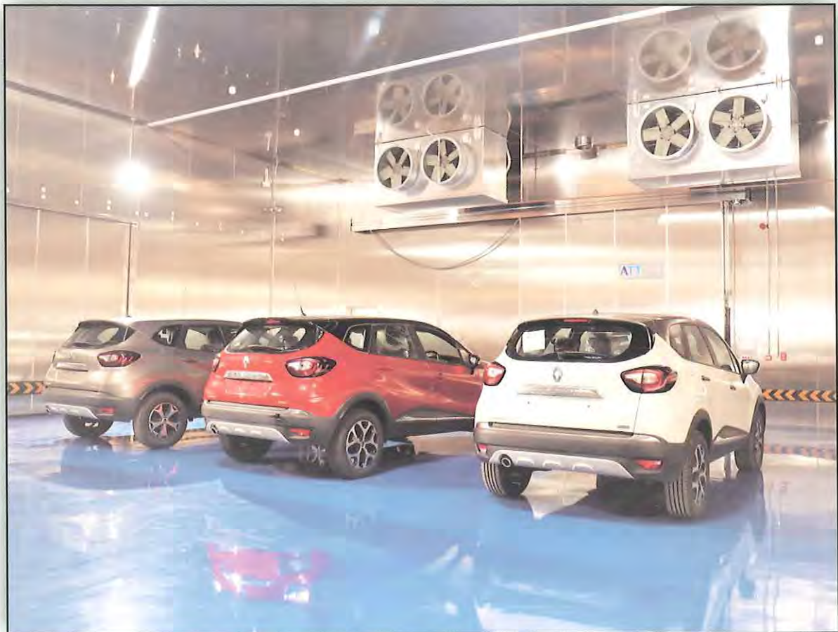
LOW TEMPERATURE SOAK ROOM AT GARC
