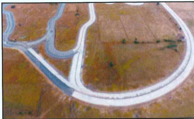
Gravel and Off road Track
