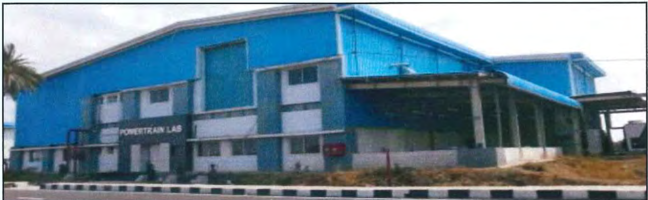
Exterior View of Power train Building
