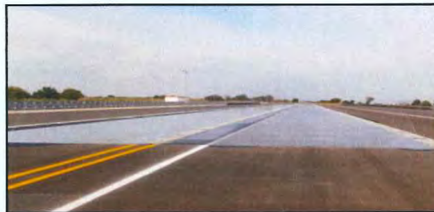
Braking Surface Track
